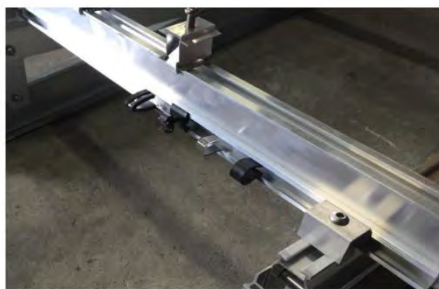
PHOTO #2: Another option for securing the PV wire to the east west rails is the optional wire management clips that TerraGen offers.
