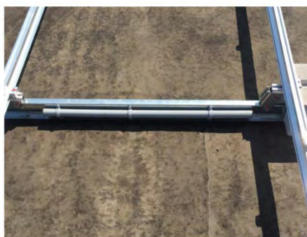
PHOTO #4: TGR base rails, (the north south rails) can be used to secure wires requiring management from row to row. We permit installers to secure wire management components to our base rail. In this case the installer used PVC conduit.
