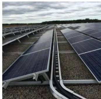
PHOTO #6: TGR base rails can be used to support cable tray for wire support running from West to East.
