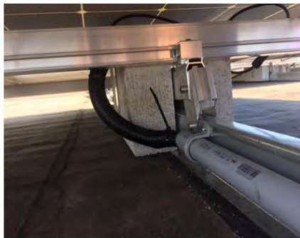
PHOTO #5: Row to row DC wiring can be pulled through PVC conduit attached to the base rail and split loom wire protection.
