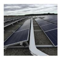
PHOTO #6: TGR base rails can be used to support cable tray for wire support running from West to East.
