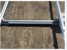
PHOTO #4: TGR base rails, (the north south rails) can be used to secure wires requiring management from row to row. We permit installers to secure wire management components to our base rail. In this case the installer used PVC conduit.
