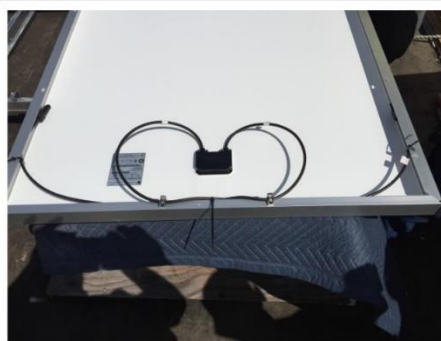
PHOTO #3: PV wire management using the optional wire management clips on the solar panel.
