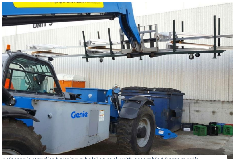
Telescopic Handler hoisting a holding rack with assembled bottom rails.
