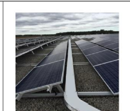
PHOTO #4: TGR base rails, (the north south rails) can be used to secure wires requiring management from row to row. We permit installers to secure wire management components to our base rail. In this case the installer used PVC conduit.
